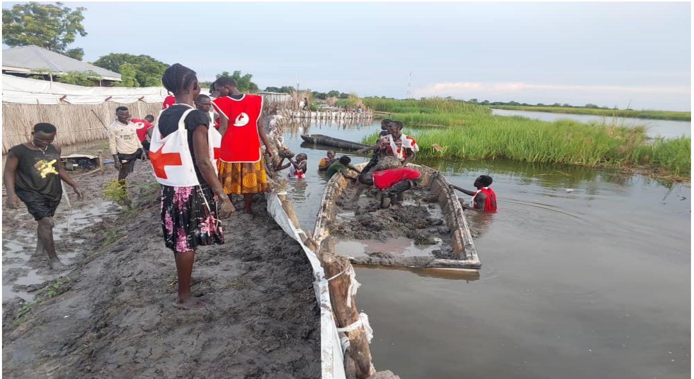
South Sudan Red Cross Volunteers repairing flood defences, (photo by SSRC)
