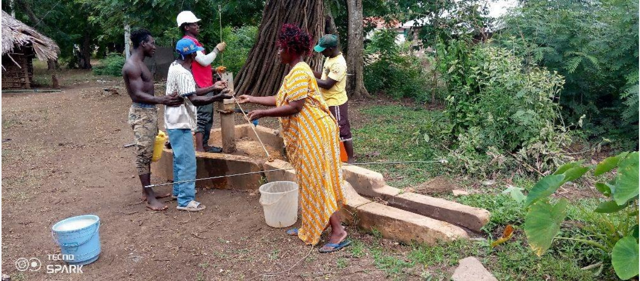
Hand pump under repair in Tana River
