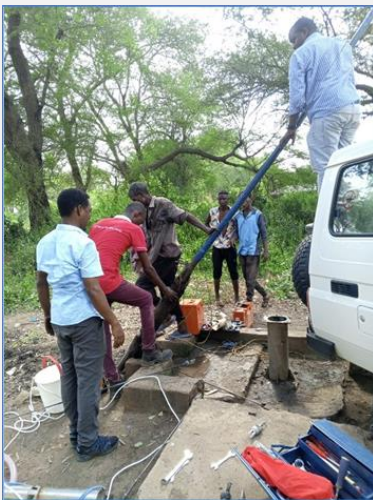
Borehole rehabilitation in Bondeni, TR County. Flushing, disinfection and replacement of pump parts. (KRCS Photo).
