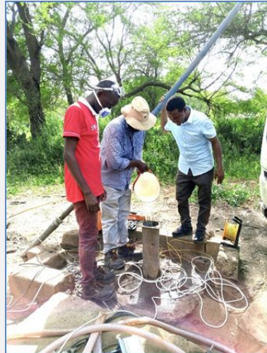
Borehole rehabilitation in Bondeni, TR County. Flushing, disinfection and replacement of pump parts. (KRCS Photo).
