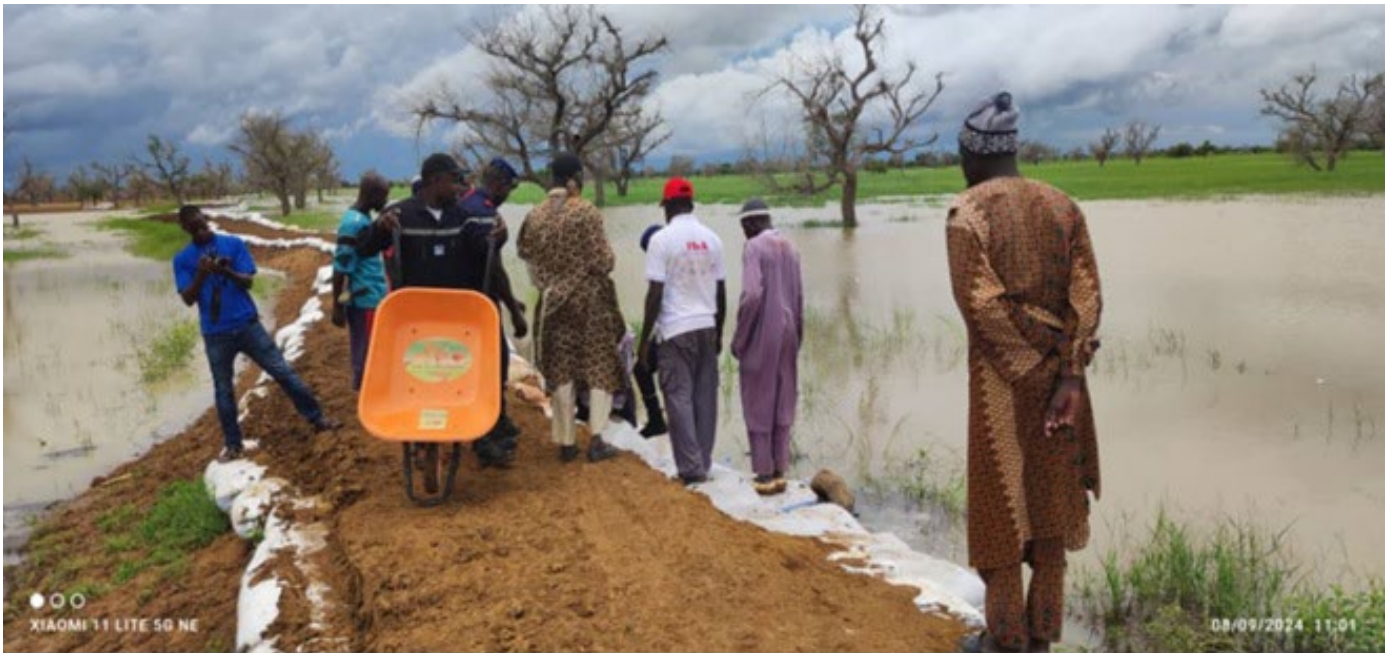
Mali Red Cross volunteers place sandbags in the Mopti region with technical services and other volunteers (Source: Mali Red Cross)
