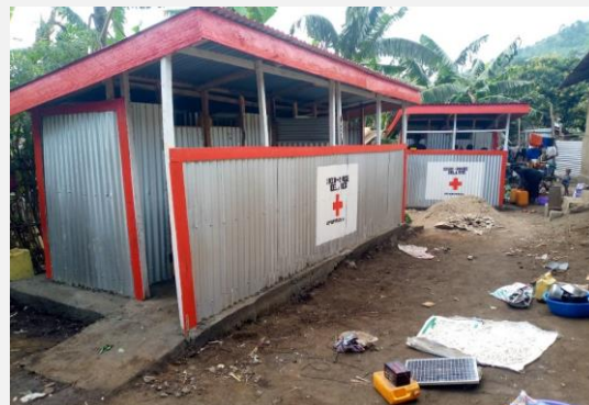
Construction of 2 blocks including: 6 emergency latrine doors and 4 shower doors in Minova
