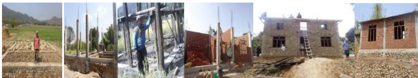
Glimpse of progress towards progressive shelter in Surkhet district. Photo: NRCS
