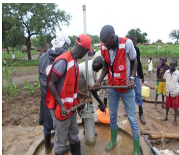
New borehole drilled and equipped. Photo: URCS
