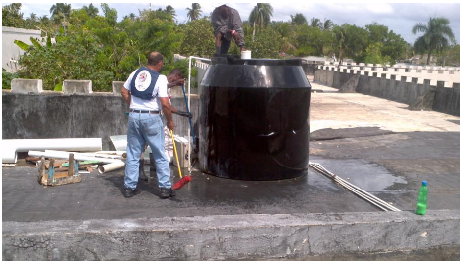
Disinfection of a water tank. Source: Dominican Red Cross
