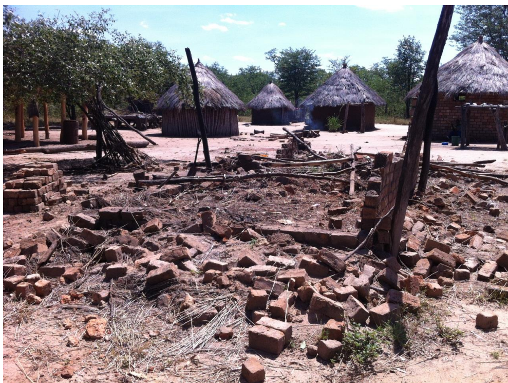
House destroyed by floods in Muzarabani District. Photo: IFRC
