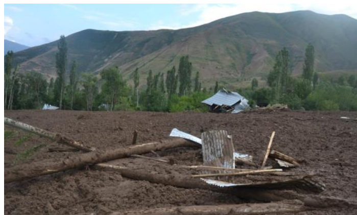
Houses are totally destroyed and left under mud in Bedak village of Rasht district. Photo: Red Crescent Society of Tajikistan
