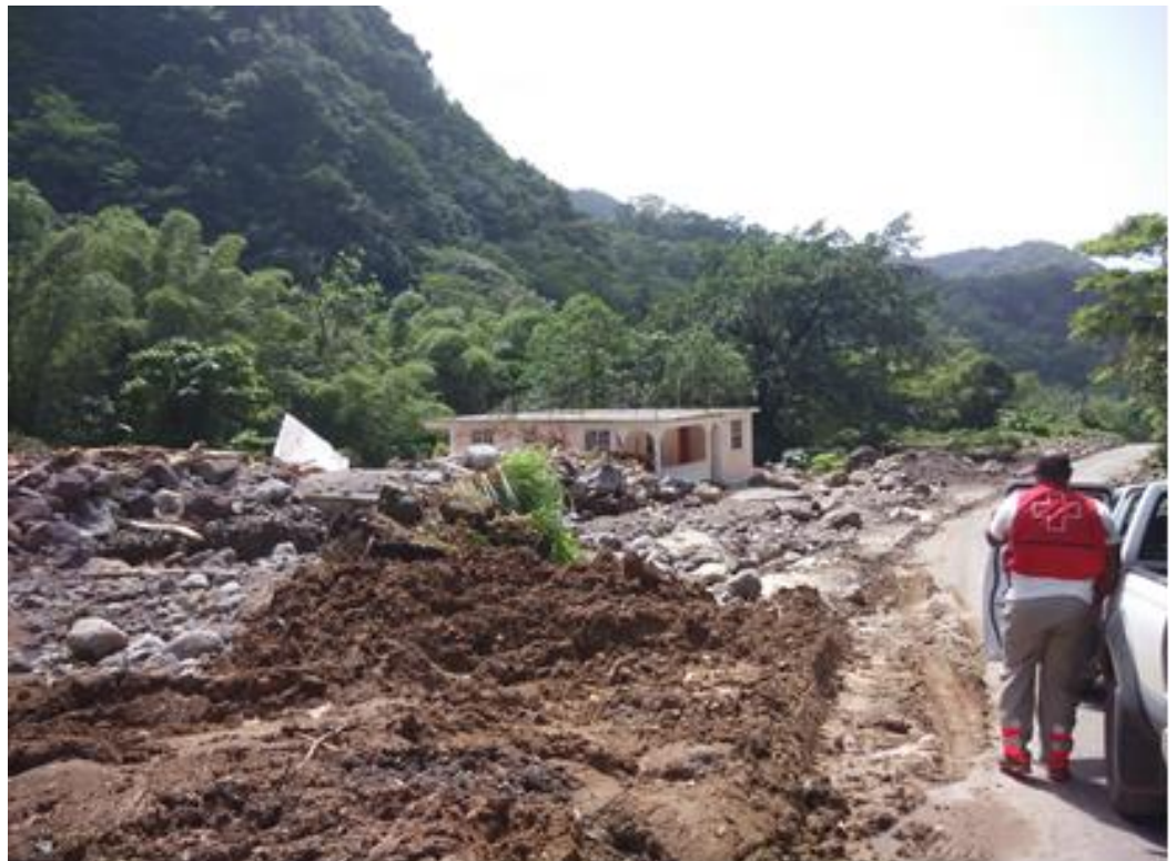
DRCS is conducted damage assessments. Source: DRCS.
