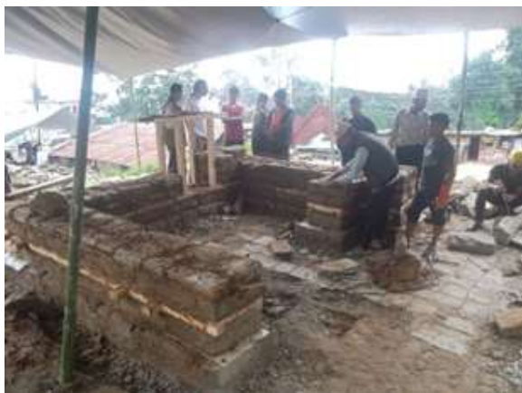
Safer construction ToT for Mason/carpenters in Dolakha. IFRC
